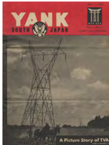
LEFT Cover of Yank: South Japan , a weekly newspaper published by the enlisted men of the U.S. Army, November 2, 1945. “This Week’s Cover: This scene shows a high-power TVA transmission line running through a Tennessee Valley rural area—symbolic of the benefits that have come from the world’s first attempt to develop an entire region.”
