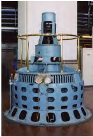
LEFT The “house generator” at Wilson Dam, 2004
